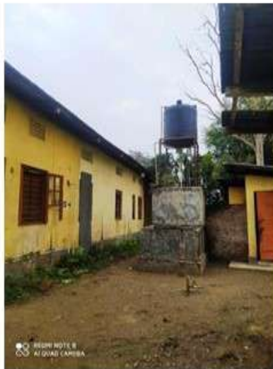
Sand water filter system
