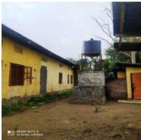
Figure 7. (a) Sand water filter system
