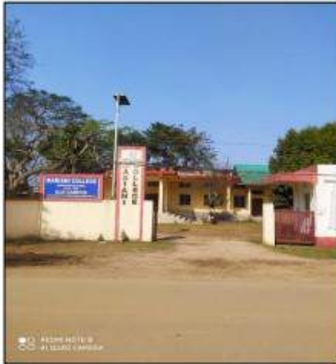
Figure 6. (a) Solar powered Street Light (Old Campus)
