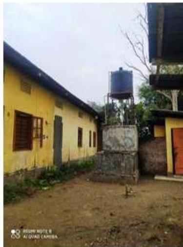
Sand water filter system
