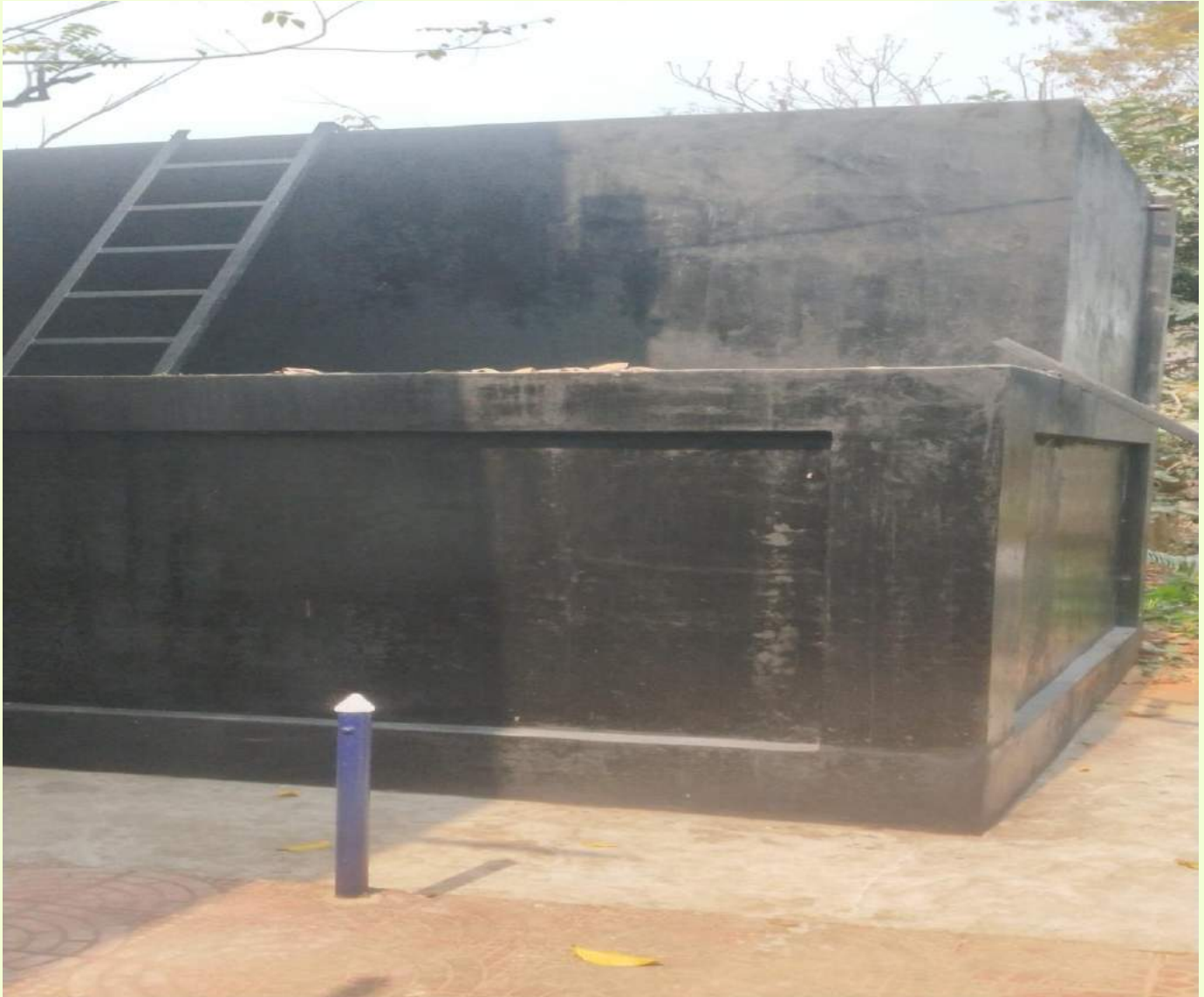
Drinking Water Plant
