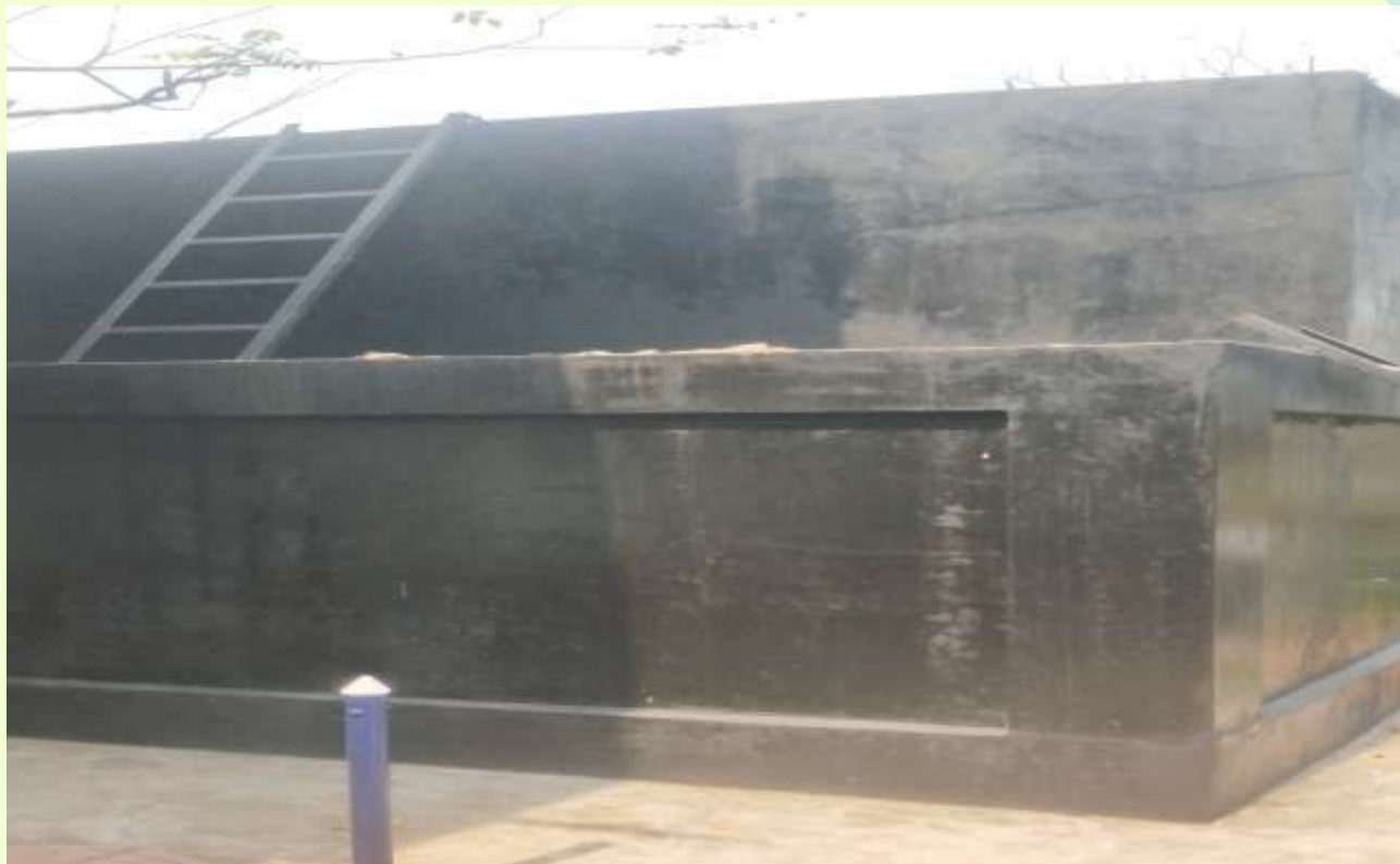
Drinking Water Plant
